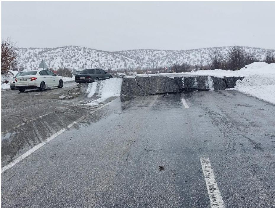
Figura 7.5. Desplazamiento lateral y vertical. (Twitter, 2023f).
